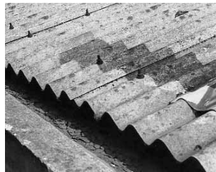
Corrugated asbestos cement roofing
